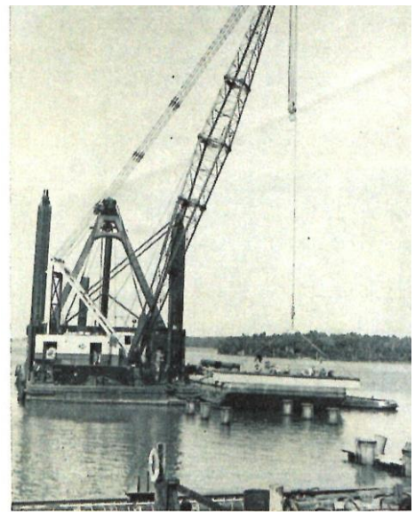
PITTS-MERRITT is 8-cu-yd diesel-electric dipper dredge.
