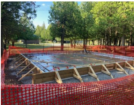
Photo (left) showing early construction with cement foundation and flooring, and photo (centre) with wall framing going up. The original concept was to adjoin the building to the pavilion, but building code requirements required the kitchen/storage facility to be a stand-alone building adjacent to the pavilion. Photo (right) shows the nearly completed exterior with kitchen facilities on the right and storage room on the left. The new building stands adjacent to the pavilion with adjoining sidewalk for ease of service access.
