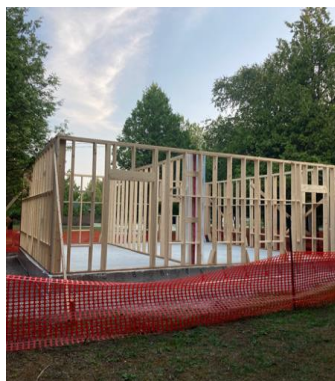
Photo (left) showing early construction with cement foundation and flooring, and photo (centre) with wall framing going up. The original concept was to adjoin the building to the pavilion, but building code requirements required the kitchen/storage facility to be a stand-alone building adjacent to the pavilion. Photo (right) shows the nearly completed exterior with kitchen facilities on the right and storage room on the left. The new building stands adjacent to the pavilion with adjoining sidewalk for ease of service access.
