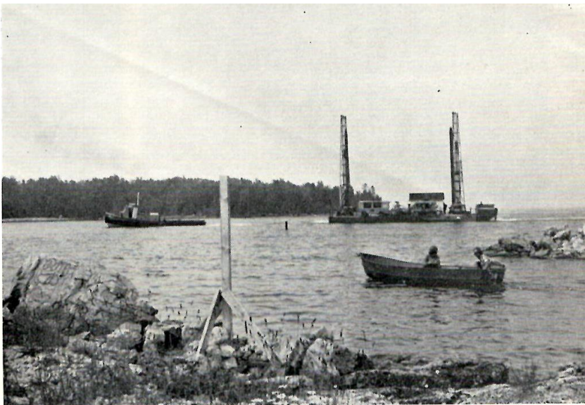
DRILLING FOR DREDGING is by Gardner-Denver 143s on barge made of unifloats.
